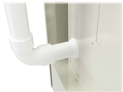
Installing vent kit through cabinet back
